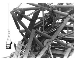
**Figure 29-1** The football stadium add-on at the University of Washington collapsed because it wasn't strong enough to support itself during construction. It likely would have been strong enough when completed, but it was constructed in the wrong order—an integration error.
