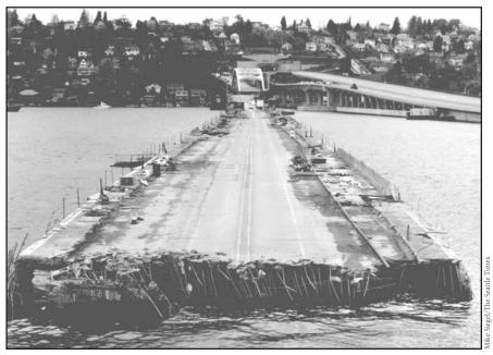
**Figure 8-1** Part of the Interstate-90 floating bridge in Seattle sank during a storm because the flotation tanks were left uncovered, they filled with water, and the bridge became too heavy to float. During construction, protecting yourself against the small stuff matters more than you might think.
